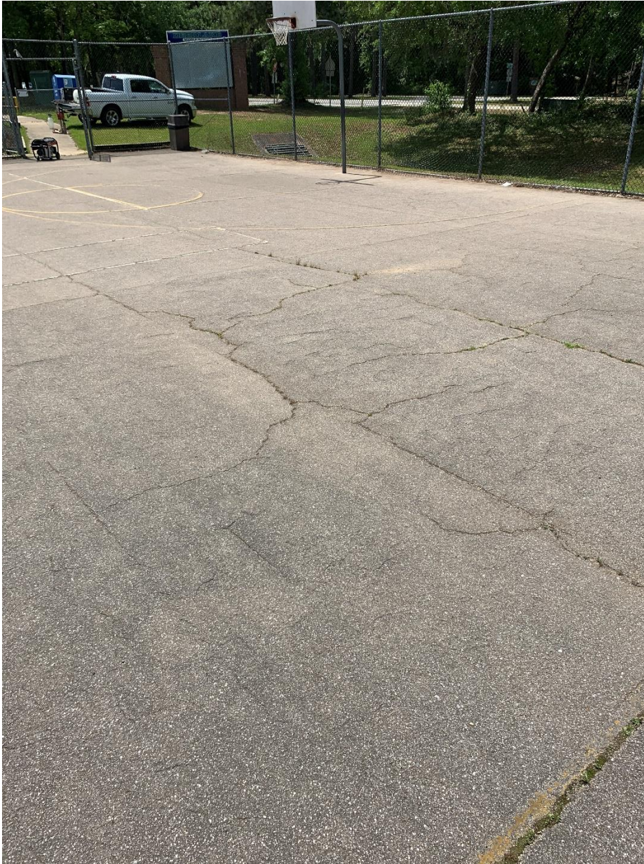
Image No. 7: Image taken at location of boring B-7, looking southwest. Image depicts intermediate to large size block cracking with isolated alligator cracking due to age. There are no visible signs of settlement in this area. The condition of the pavement in this area of the courts is fair.
