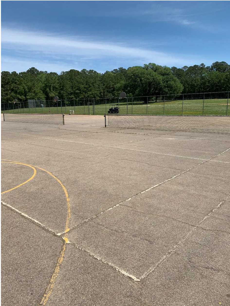
Image No. 8: Image taken at location of boring B-8, looking northeast. Image depicts intermediate to large size block cracking due to age. There are no visible signs of settlement in this quadrant. The condition of the pavement in this area of the courts is fair.
